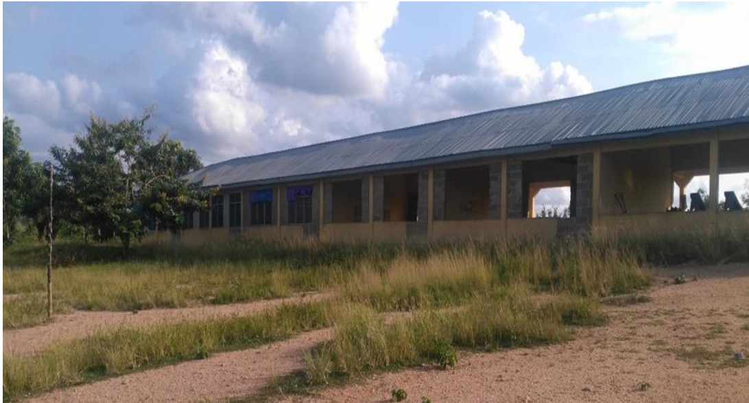
Pic. A. Six Classroom Pavilion at Bawjiase SHS. (Awutu Senya District)
