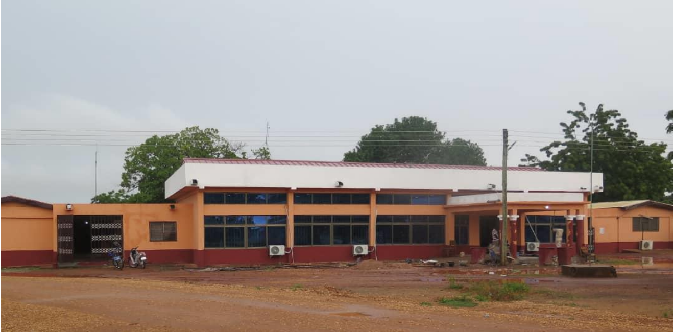
Renovated Saboba District Assembly Hall
