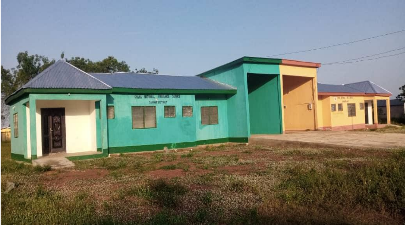
Newly Constructed Fire and Ambulance Stations
