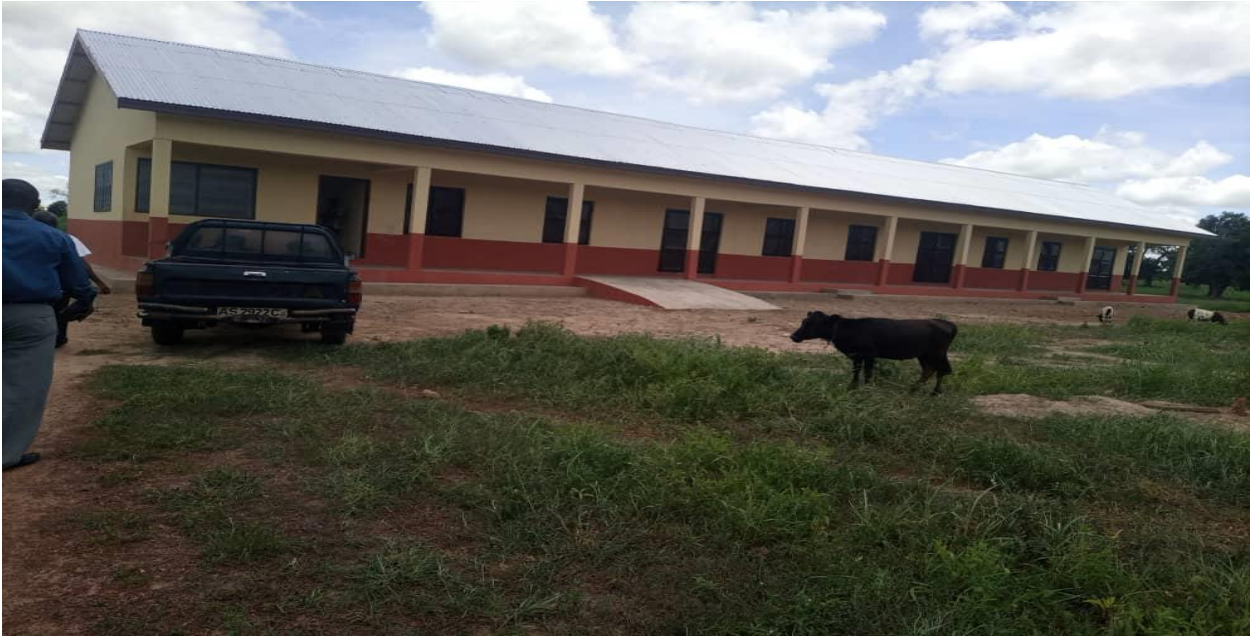
Completion of a 3-unit Classroom block at Zambo Kokori
