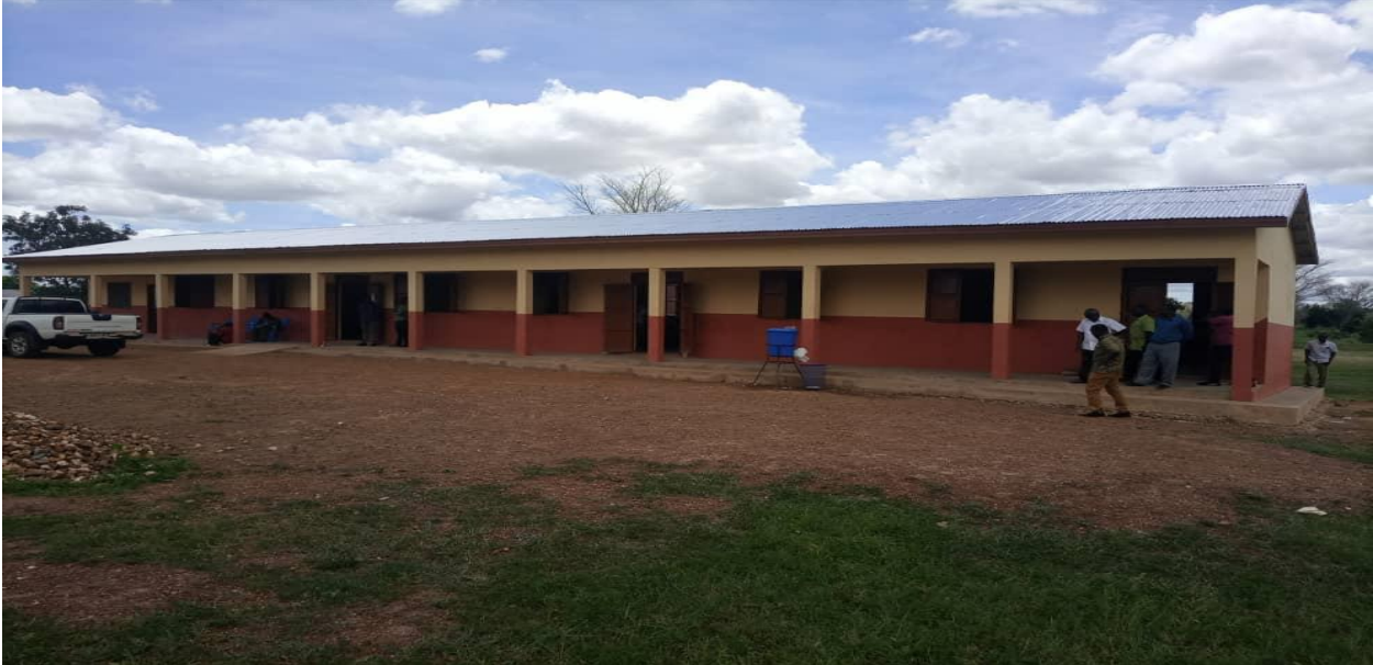
Completion of a 3-unit Classroom block at Tampie
